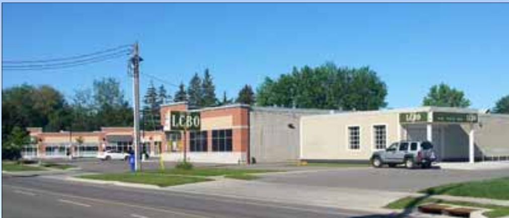
LCBO neighbour foreground, Subject plaza background
